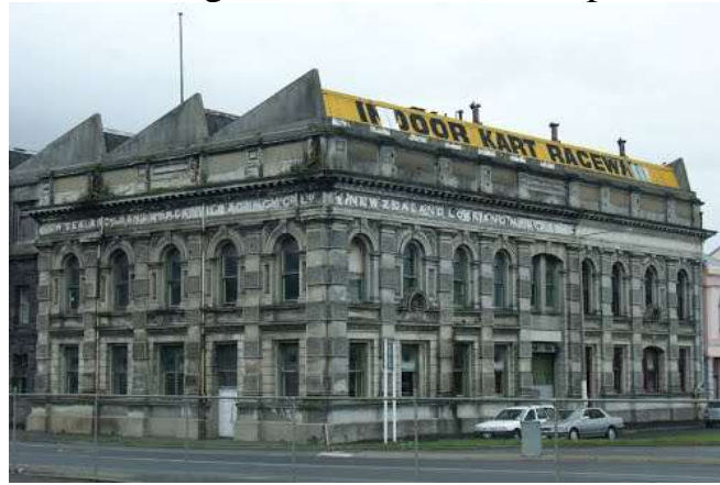
Stewarts Building Thomas Burns St. Top Floor 1991
